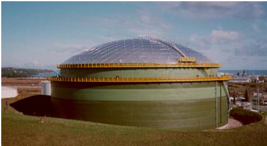
Figure 1. Gasoline tank in Sermin near Koper, Slovenia made from the steel Niomol 490 K.
